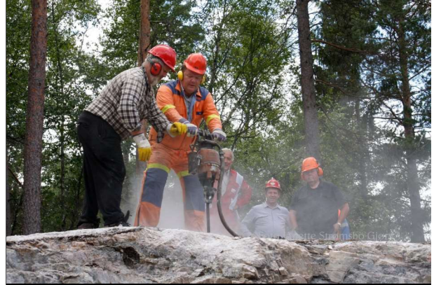
County governor Djupedal drilling a hole in the Steli mine
